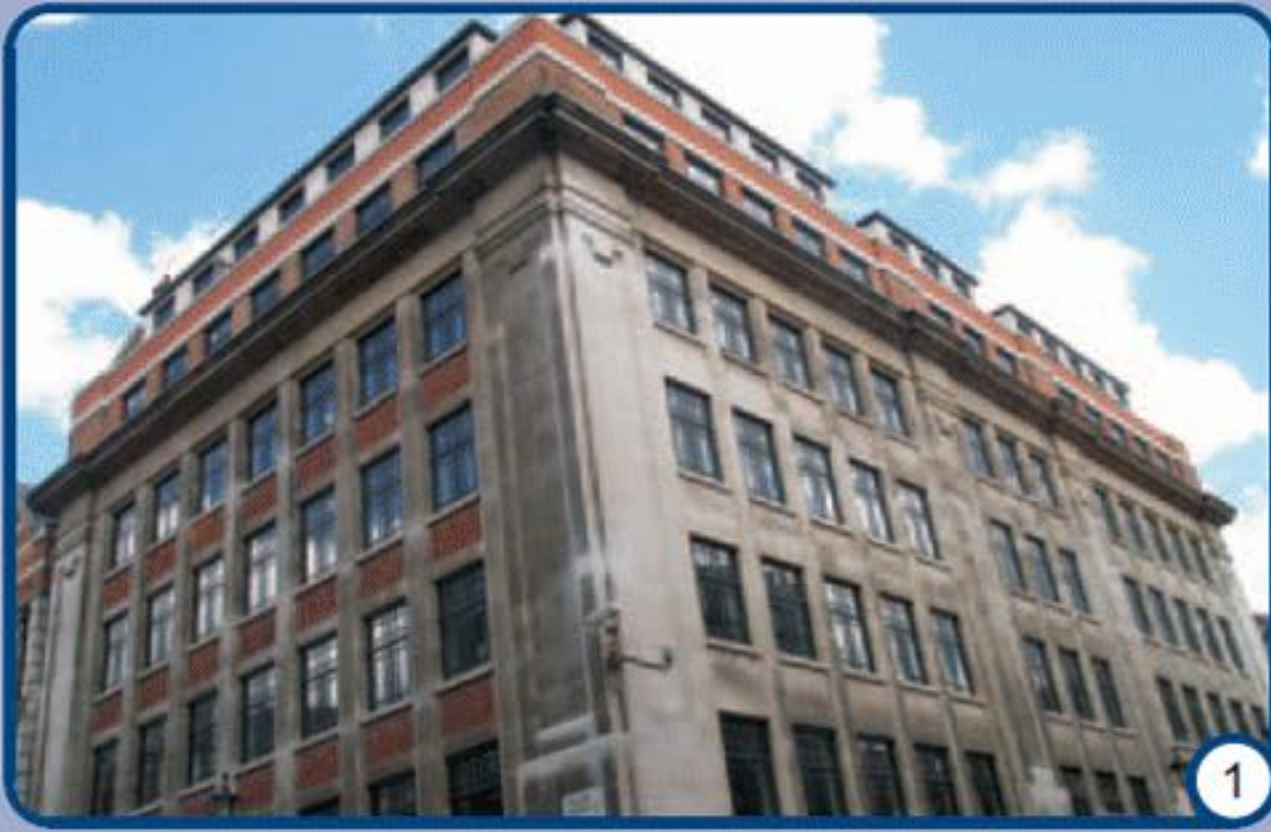
1. W40 replacement double glazed blast-resistant black powder steel windows in central London commercial building
