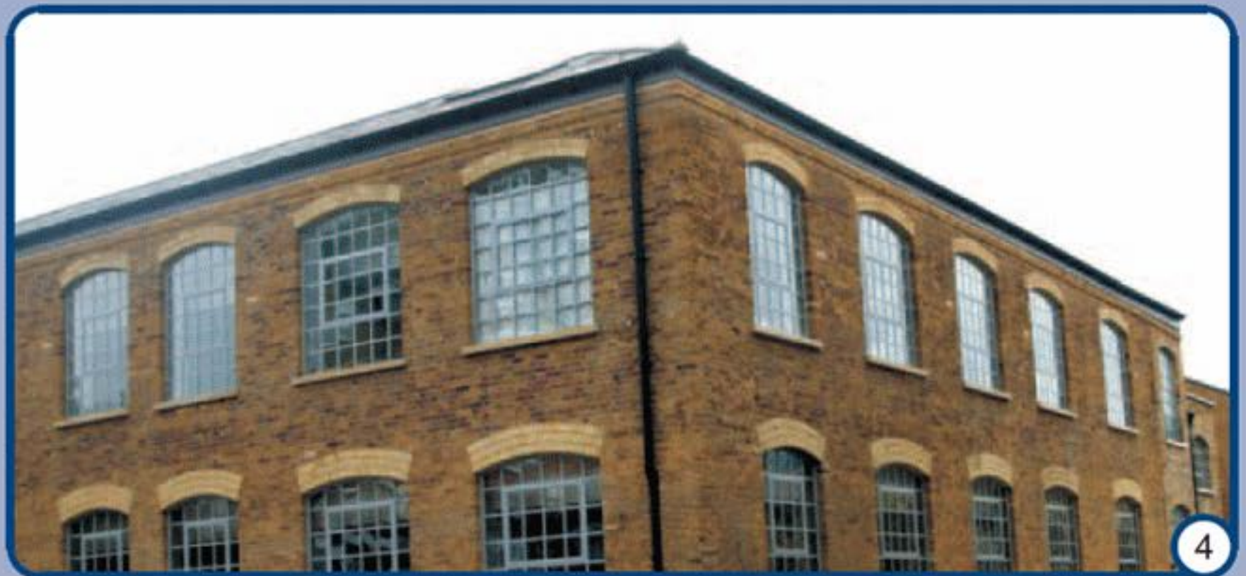
4. W20 series galvanised and polyester powder coated double glazed windows with true steel glazing bars retain the aesthetic but increase thermal insulation in a London warehouse conversion project
