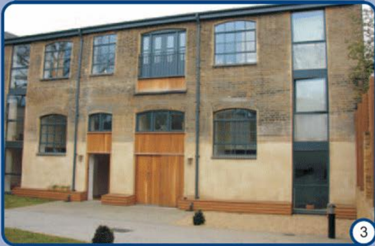
3. W20 dark grey polyester powder coated double glazed windows and doors used in a variety of styles on a North London conversion
